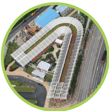
Administration Building 行政大樓
